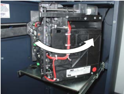
Rotate mechanism to operate position (counterclockwise).
